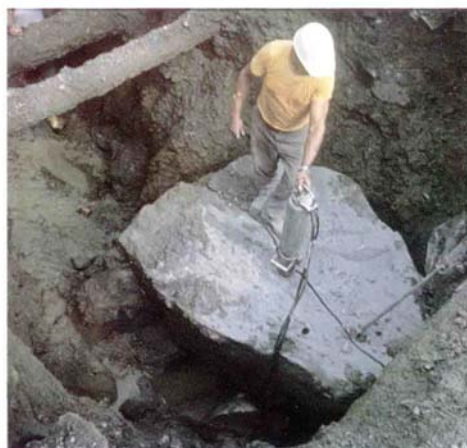
Trench rock and boulders below grade can be broken with one or more hydraulic splitters. Hydraulic splitting eliminates dangers associated with blasting. These hydraulic splitters will also operate underwater without any modifications.
