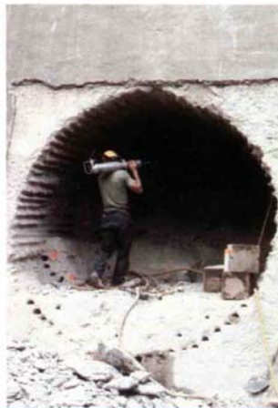
Left, Hydraulic splitter was used to remove ends of overpass supports to form a keyway. The concrete was separated wide enough to cut reinforcing rods using enlarging feathers. Right, Workman carries splitter used to cut 14 ft. tunnel through base of dam for new penstock.
