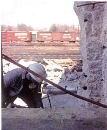
Left, Hydraulic splitter was used to remove ends of overpass supports to form a keyway. The concrete was separated wide enough to cut reinforcing rods using enlarging feathers. Right, Workman carries splitter used to cut 14 ft. tunnel through base of dam for new penstock.
